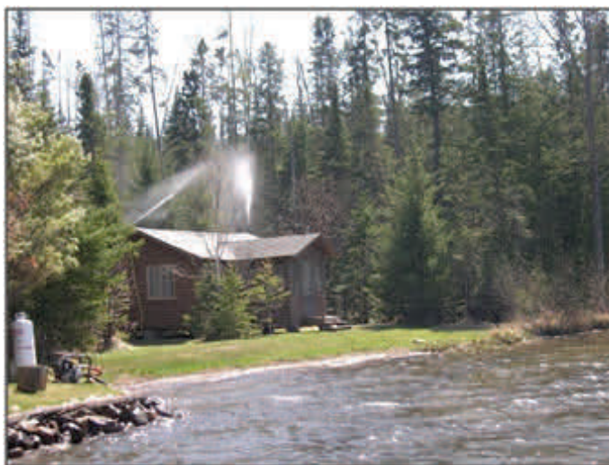
House sprinkler system in Minnesota. Credit: Northeast Region
