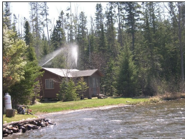
Image 3 Sprinkler system at private residence in Minnesota
